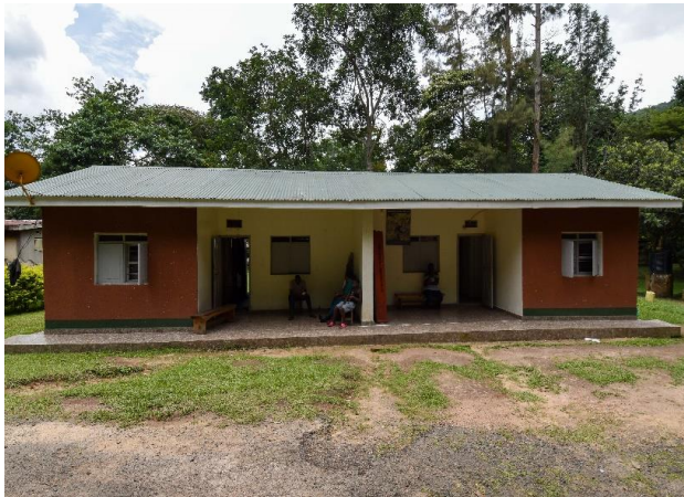
Staff house at Kalinzu sector to be renovated
