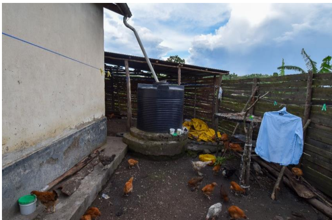
Tank Stand to be demolished and reconstructed at Kalinzu Beat
