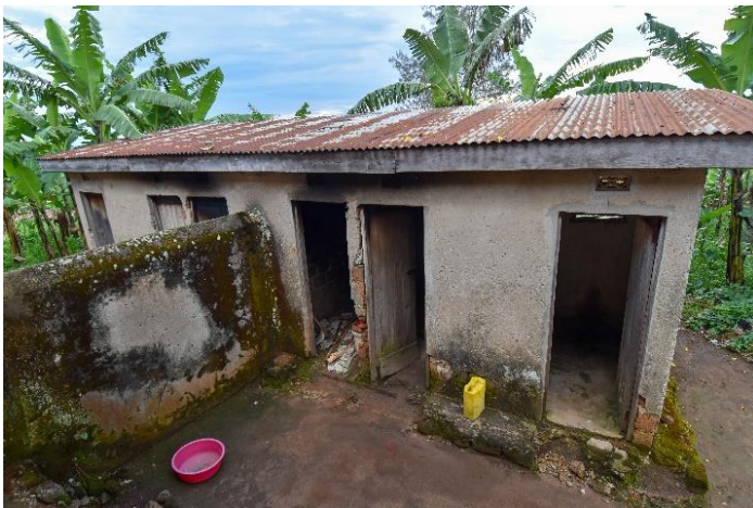
Store house to be renovated at bitereko
