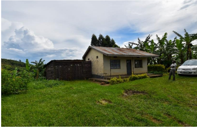
Kalinzu beat office to be renovated
