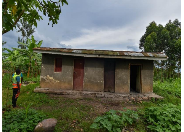
Staff house store at Kalinzu beat to be renovated
