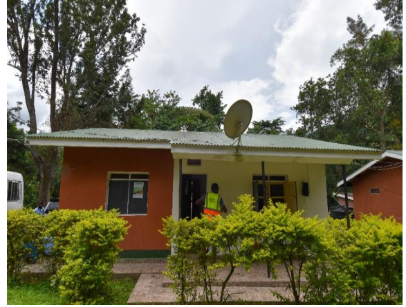
Kalinzu Sector Office to be renovated
